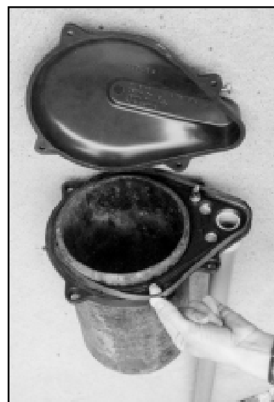
Figure 5.2.9b. Well Cap with Vent
